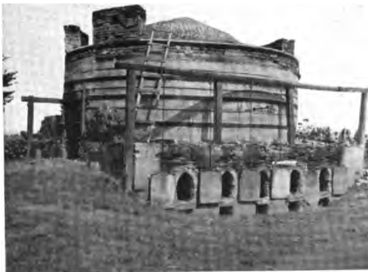
(B) Kiln at Stevensburg brick plant.
